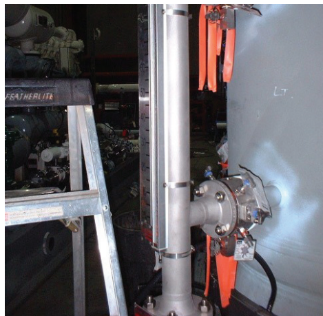
A bridle with Parker monoflanges for low viscosity fluids. Note the capillary leading to instrument transmitter.
