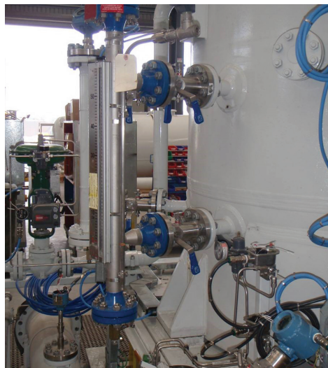
A bridle with Parker monoflanges for low viscosity fluids. Note the capillary leading to instrument transmitter.
